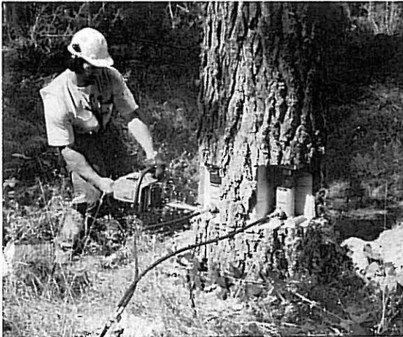
*Figure 2 - Saw operator completing split level cuts*
