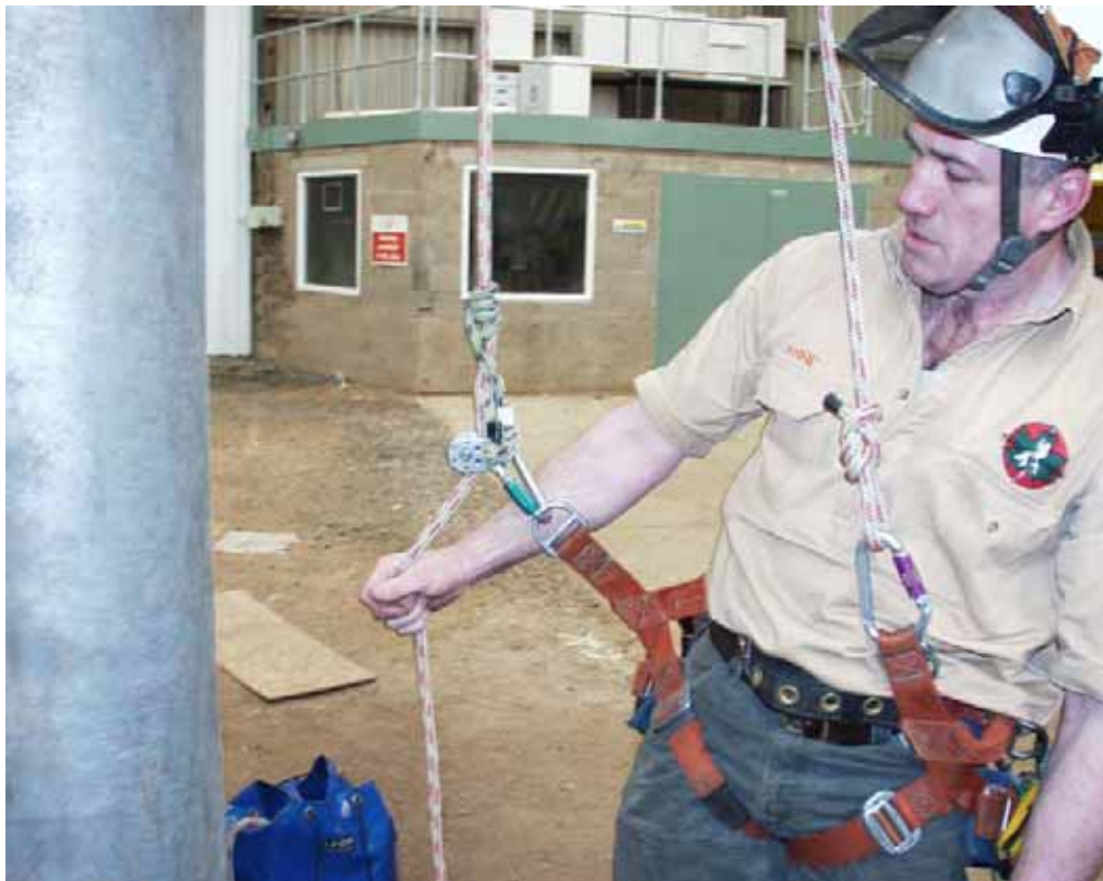
Figure 13 – Use of pulley on support rope.
