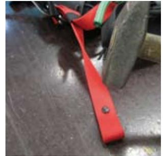
12. Place the strap on a solid surface, and use a hammer to drive the rivet into place.
