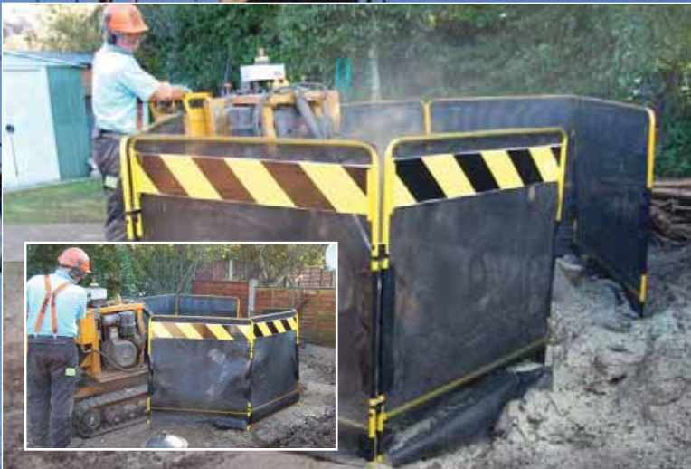
The Modular Guarding System is designed to help reduce the risk of flying debris and helps to protect your customer's property from damage.
