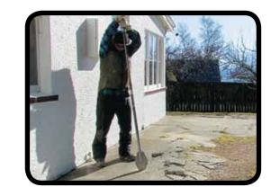
TIP: THE SLAMMER TOOL IS GREAT FOR PUTTING IN PILOT HOLES FOR WOODEN PEGS FOR BOXING (AND FOR GETTING THEM OUT WITHOUT BREAKING THEM) AND ALSO FOR REMOVING THE BOXING.
